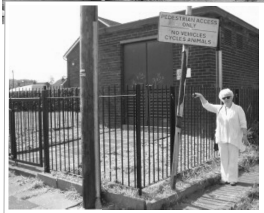
Councillor Jane Gartside at Brimrod Sub-Station before and after the clean-up
